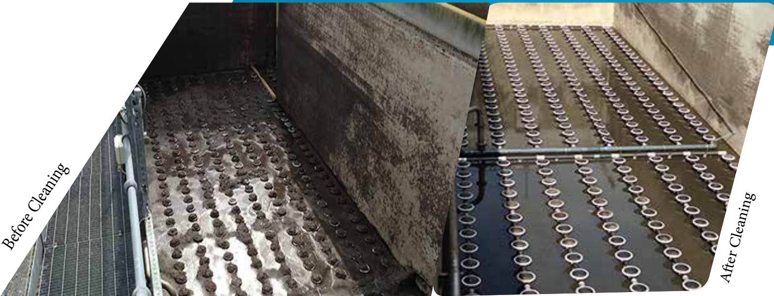
2.5 TANK CLEANING, DE-MUCKING & DE-SLOPING
